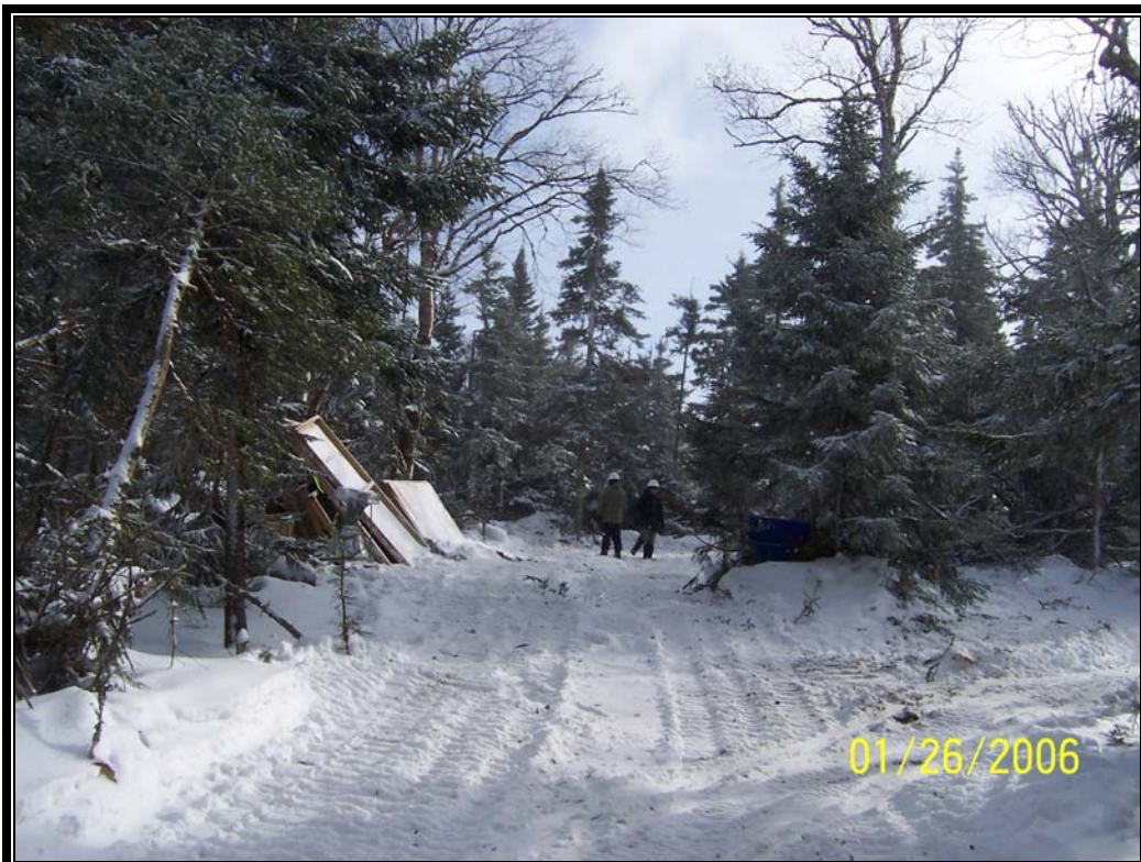
View southeast of A1 tower location (where workers are standing) from access trail.
