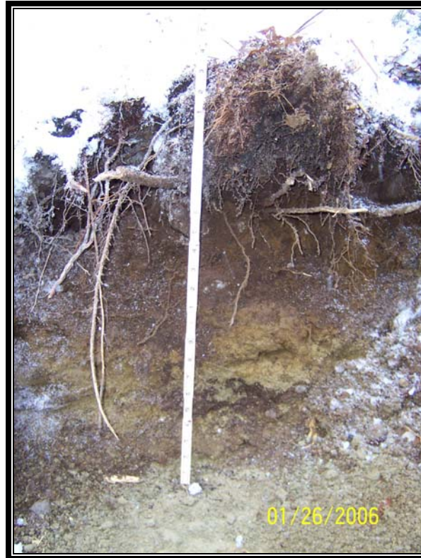
Test Pit TP-A1 SA (south anchor) western side wall.
