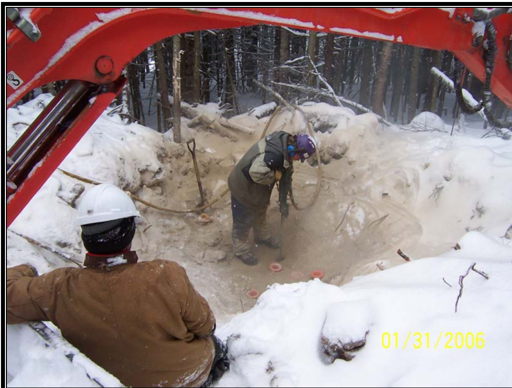
Manually operated jack hammer drilling at A1 NA (north anchor).
